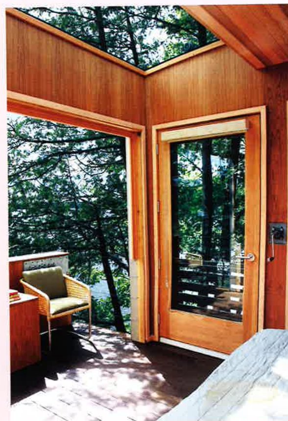
THE MOVING FLOOR SLIDES OUT TO CREATE AN OPEN-AIR SITTING AREA.
