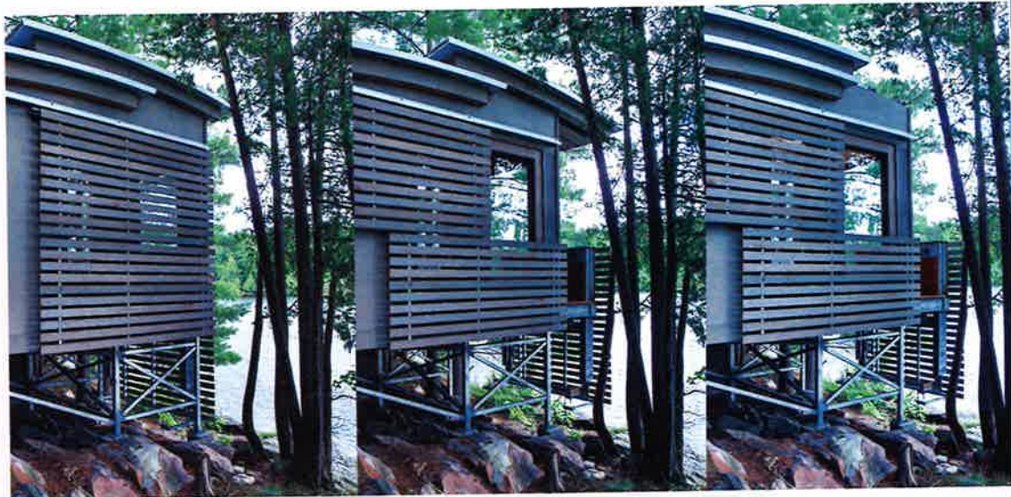
LIKE THE OLD BUNKIE, THE NEW ONE SITS ON STILTS, WHICH ALLOWS RAINWATER TO BE DIRECTED DOWN TO THE LAKE.
